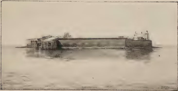
FORT SUMTER, AS REBUILT
