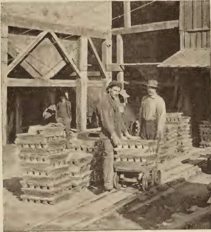
BULLION AT THE AMERICAN SMELTER, LEADVILLE, COLORADO
