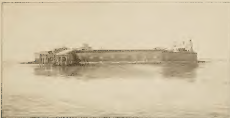
FORT SUMTER, AS REBUILT
