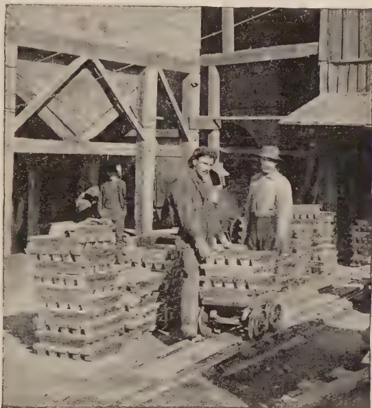
BULLION AT THE AMERICAN SMELTER, LEADVILLE, COLORADO
