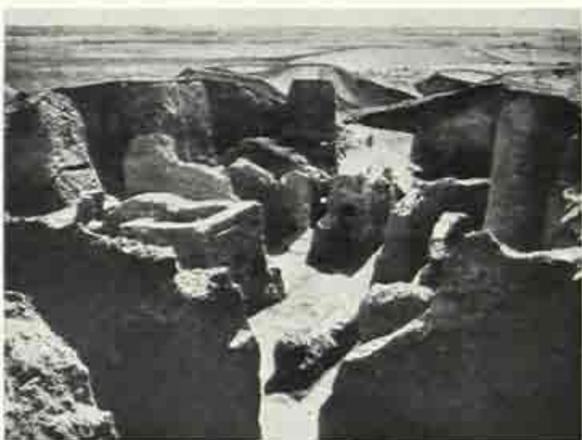
1. Ruined temple-library at Nippur
