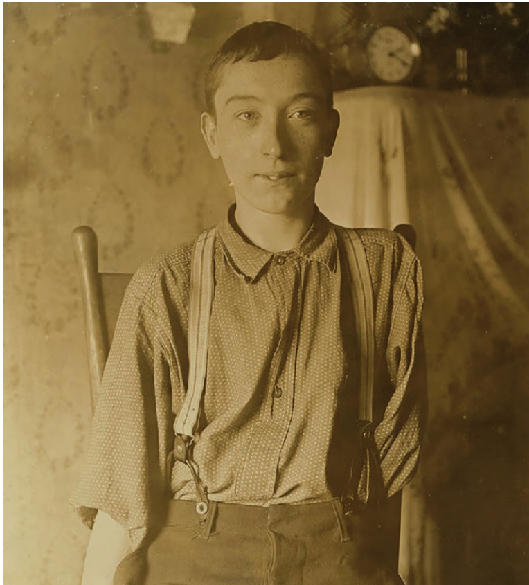
Figure 6.3 Harry McShane, who celebrated his sixteenth birthday a month or so before this photo was taken by social reformer and photographer Lewis Wickes Hine, lost his left arm as a result of a workplace injury in May 1908 in Cincinnati, Ohio. McShane had already been working in the factory for more than two years. Before federal safety regulations (such as OSHA and FLSA), catastrophic injuries on the job were common, as was the presence of children in the workforce. McShane received no compensation for his injuries. (credit: modification of "Lewis Wickes Hines - Harry McShane 1908" by "Fordmadoxfraud"/Wikimedia Commons, Public Domain)
